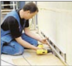
5 Fastening of lower start profile.
