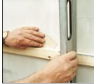
2 Adjusting surface alignment by inserting spacers behind the battens.
