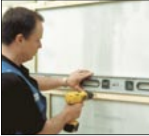
1 Putting up battens behind the panels.
