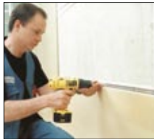
6 Screwing in the joint profile.
