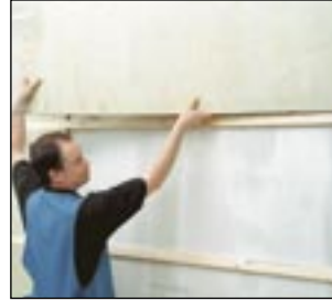
3 Inserting mineral wool slabs between battens.
