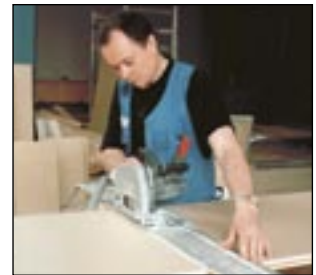
8 Sawing the panel from the back. Use tools with extraction facilities.
